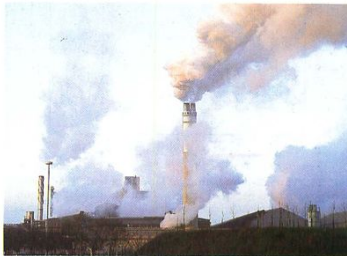
Fig. 21 Air pollution by industry. Tall chimneys keep pollution away from the immediate surroundings but the atmosphere is still polluted.
